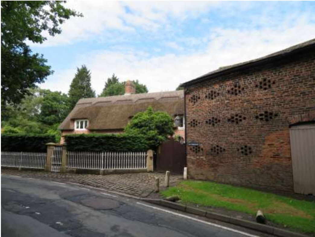
Plate 1 Davenport Green Farmhouse and Barn. Paddy's Hut sits within the private residential plot and is not visible from the road
